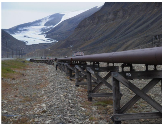
Overground pipe in Longyearbyen.
