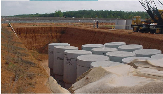
Low level nuclear waste disposal in buried drums (nrc.gov).
