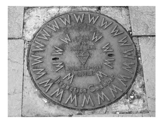
(a) The cover is marked 'ductile'. It is made from ductile iron, which was invented in 1943. It replaced the previous form of cast iron, which was more brittle.
