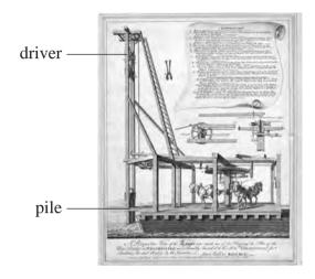
(a) (i) The driver on the pile driver above had a mass of 810 kg and could be dropped a maximum distance of 6.0 m onto the pile.
