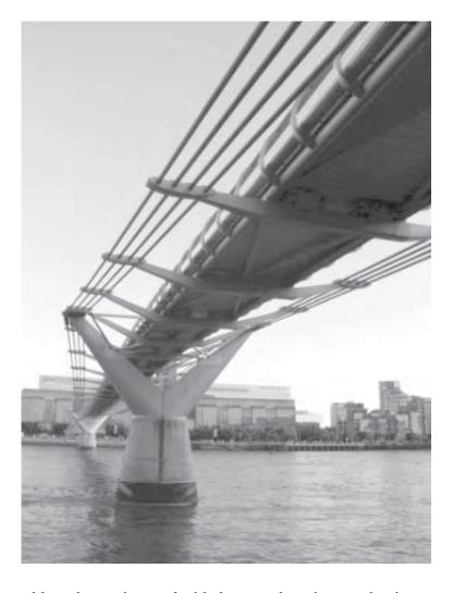
To solve the problem the engineers decided to use damping mechanisms – giant shock absorbers to limit the bridge's response to external forces. They decided to use two systems: viscous dampers, similar to car shock absorbers, and tuned mass dampers. A tuned mass damper is a large mass stiffened by springs.
