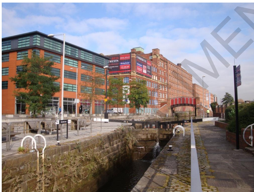
A modern photograph of the former cotton mills and Rochdale Canal, Redhill Street.
