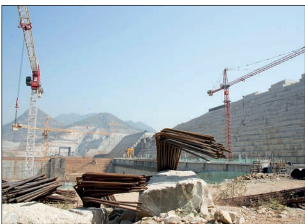
The construction site of the dam
