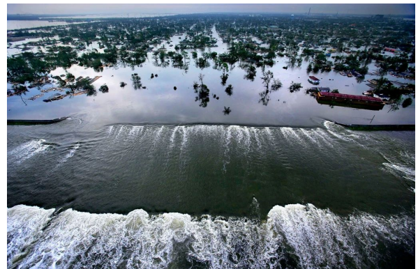
A failed levee in New Orleans after Hurricane Katrina. (Source: www.nytimes.com )
