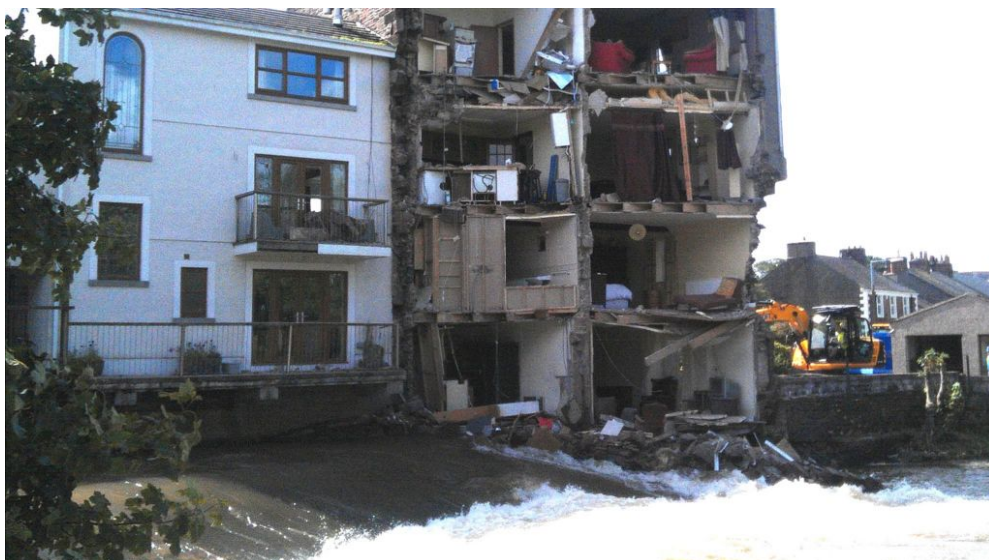
A house falls into a river by the River Ehen in Cumbria after heavy rain triggered mass movement.
