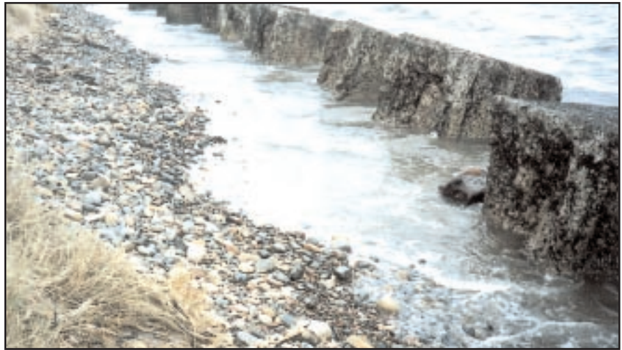
Figure 1: Human or physical influences? WW2 tank traps on a Northumbrian beach protect sand dunes from erosion at high tide.
