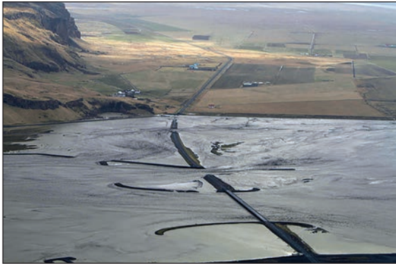
Figure 5b: Highway 1, the road that goes around Iceland, is cut off by a flood
