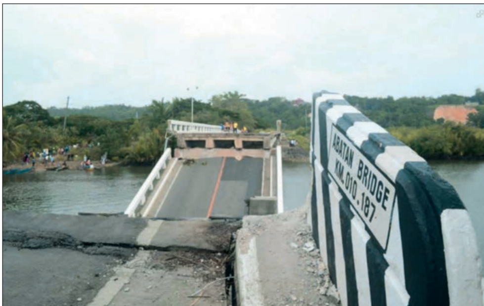
Figure 6d: The destroyed Abatan Bridge that connects Maribojoc to Tagbilaran City, the capital of Bohol
