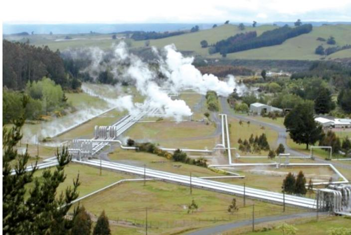
Hot rock under the surface of the earth can heat water converting it to steam. This then generates electricity in the same way as coal, oil, gas or nuclear powered stations.
