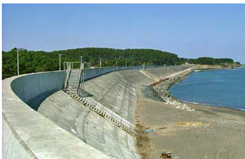
Ibaraki – a 10m high tsunami wall protecting low lying areas
