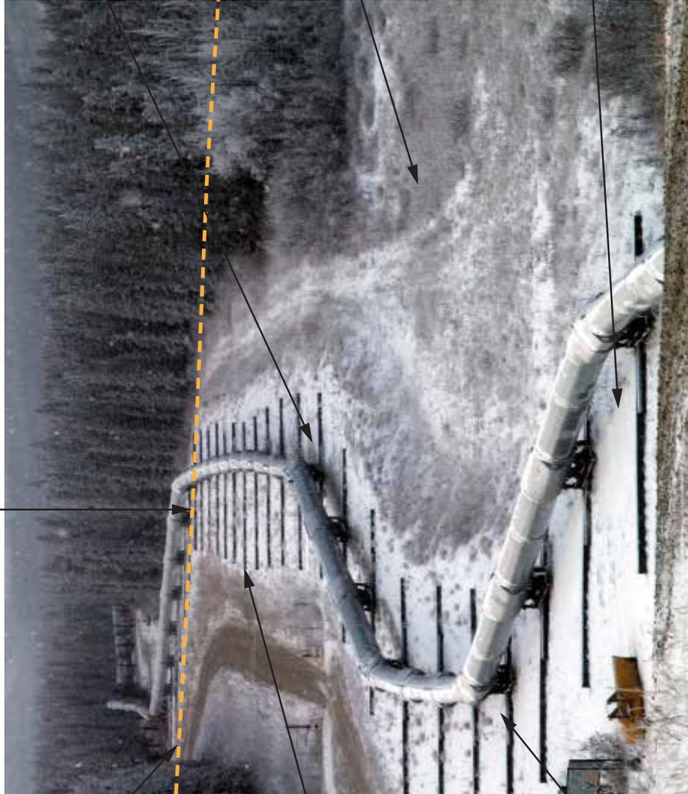
Insulated supports prevent permafrost thaw and solifluction caused by heated oil
