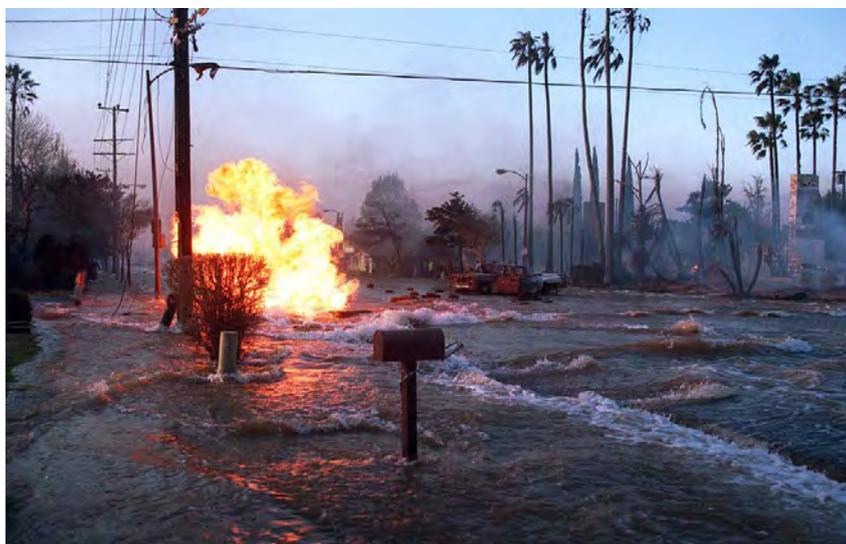
Gas from a ruptured supply line burns as water from broken water main floods Balboa Boulevard in the Granada Hills area of Los Angeles, on January 17, 1994. The fire from the gas main destroyed two homes.
