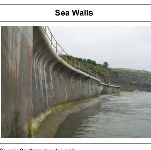
Source: Southampton University Description: Concrete structures that absorb and reflect wave energy, with curved surface Effective erosion prevention
