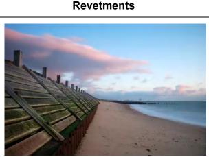
Source: Geographical.co.uk Description: Wooden or concrete ramps that help absorb wave energy
