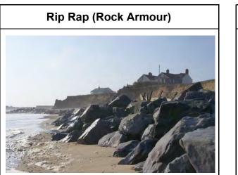
Source: Stacey.Peak-Media Description: Large rocks that reduce wave energy, but allow water to flow through Cost effective
