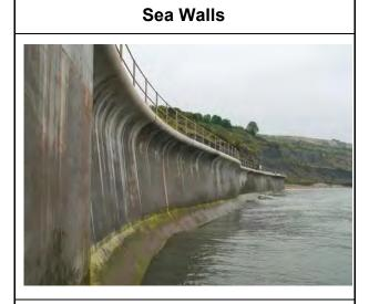
Source: Southampton University Description: Concrete structures that absorb and reflect wave energy, with curved surface Effective erosion prevention
