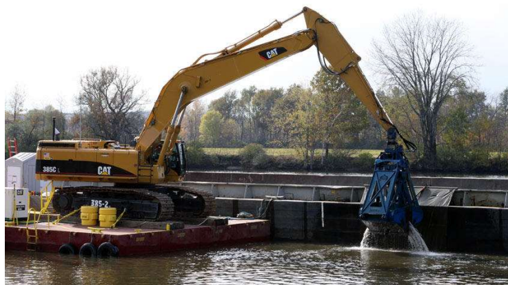
Dredging in the Hudson River. Source: EPA.
