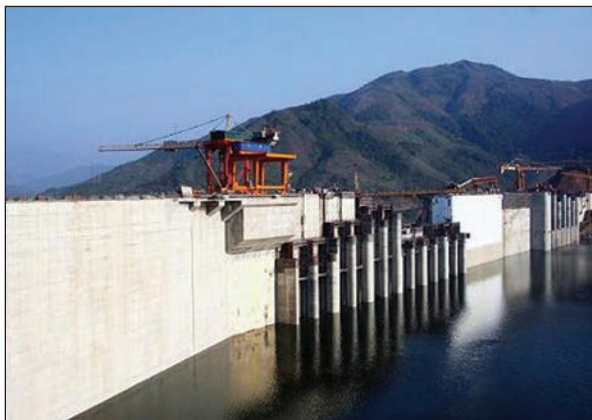
HEP station under construction in Vietnam
