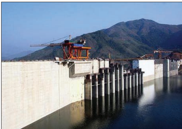
HEP station under construction in Vietnam
