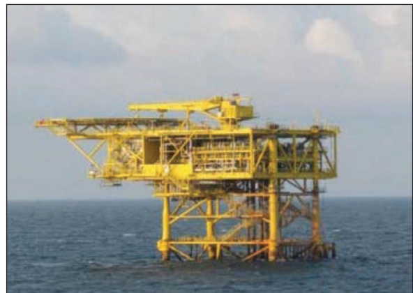
Gas platform off the coast of Vietnam
